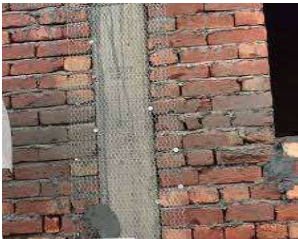
(Classic Fib Mesh100 used for Electrical Pipe Plastering)
